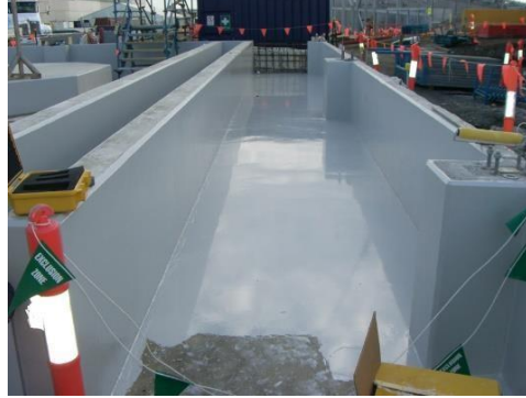
Concrete Protective Coating
