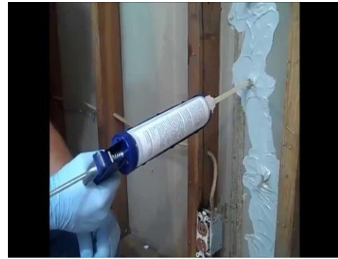
Concrete Crack Repair with PU Injection Method
